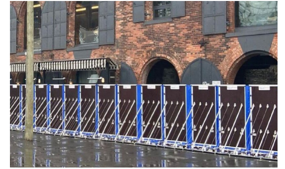
The Deployable Flood Shield System Protecting the Empire Stores. Source: Twitter Posting of AquaFence.
